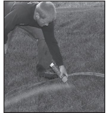
Fig. 1 Spray paint and outline the shape.
