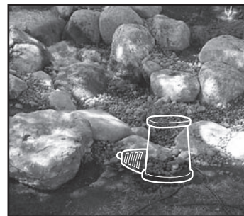
Fig. 22 Set larger boulders (6" – 18") around the perimeter of the basin.
