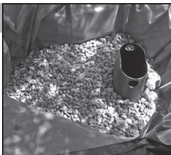
Fig. 21 Add the 1 1/2" to 2" size gravel.
